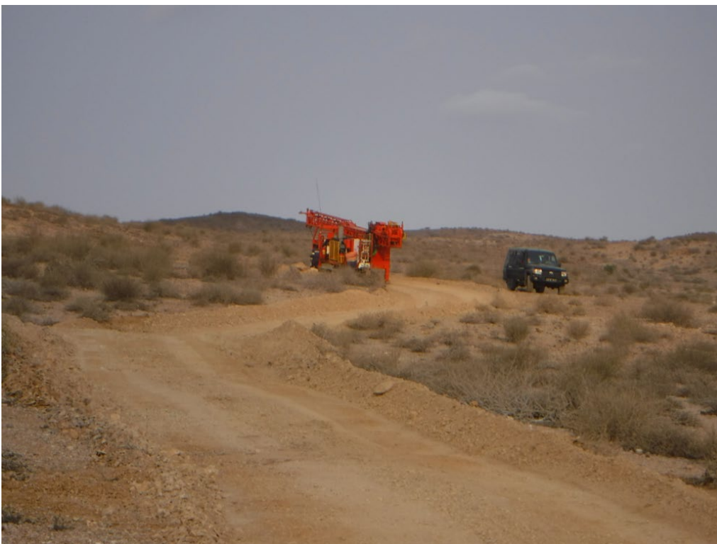
Figure 2: Geoangol (drilling contractor) drill-rig tramping along repaired access track towards drill-site.
