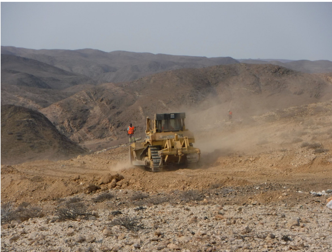
Figure 4: Preparation of drill-pad for the first drill-hole at Muvero Prospect.
