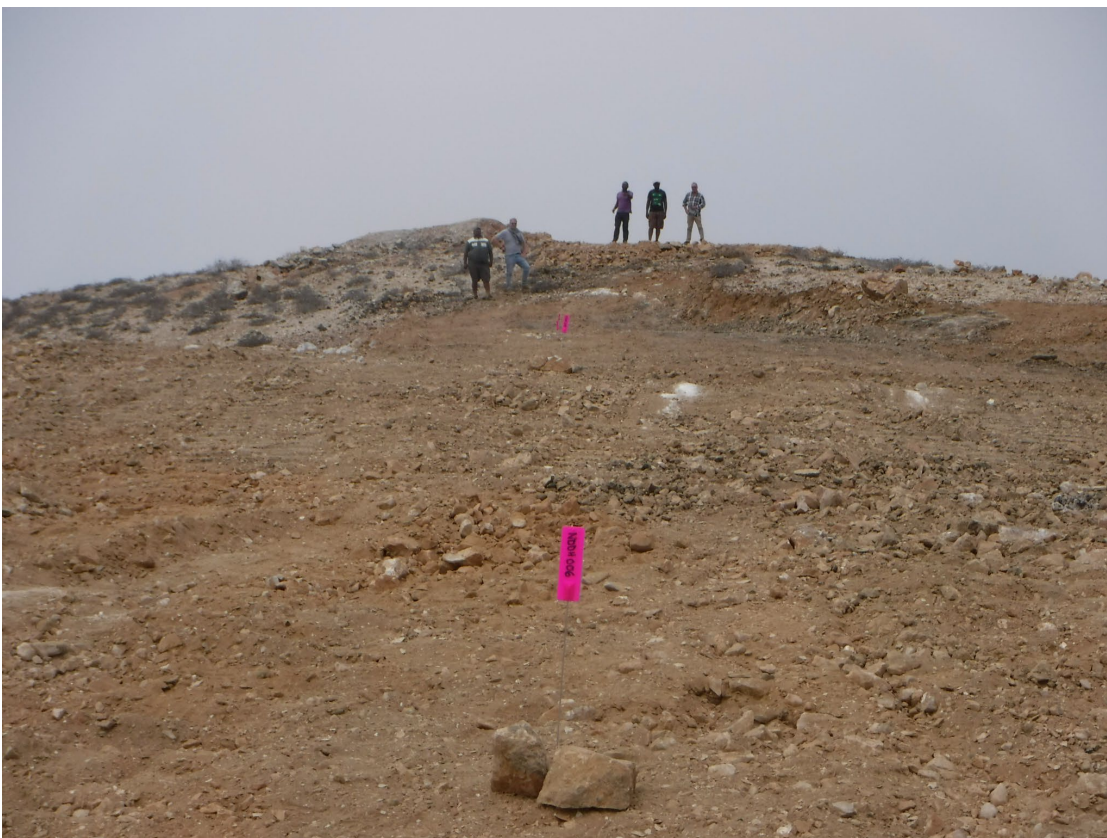
Figure 6: Marked-out drill-collar locations, shown by pink pin-markers.
