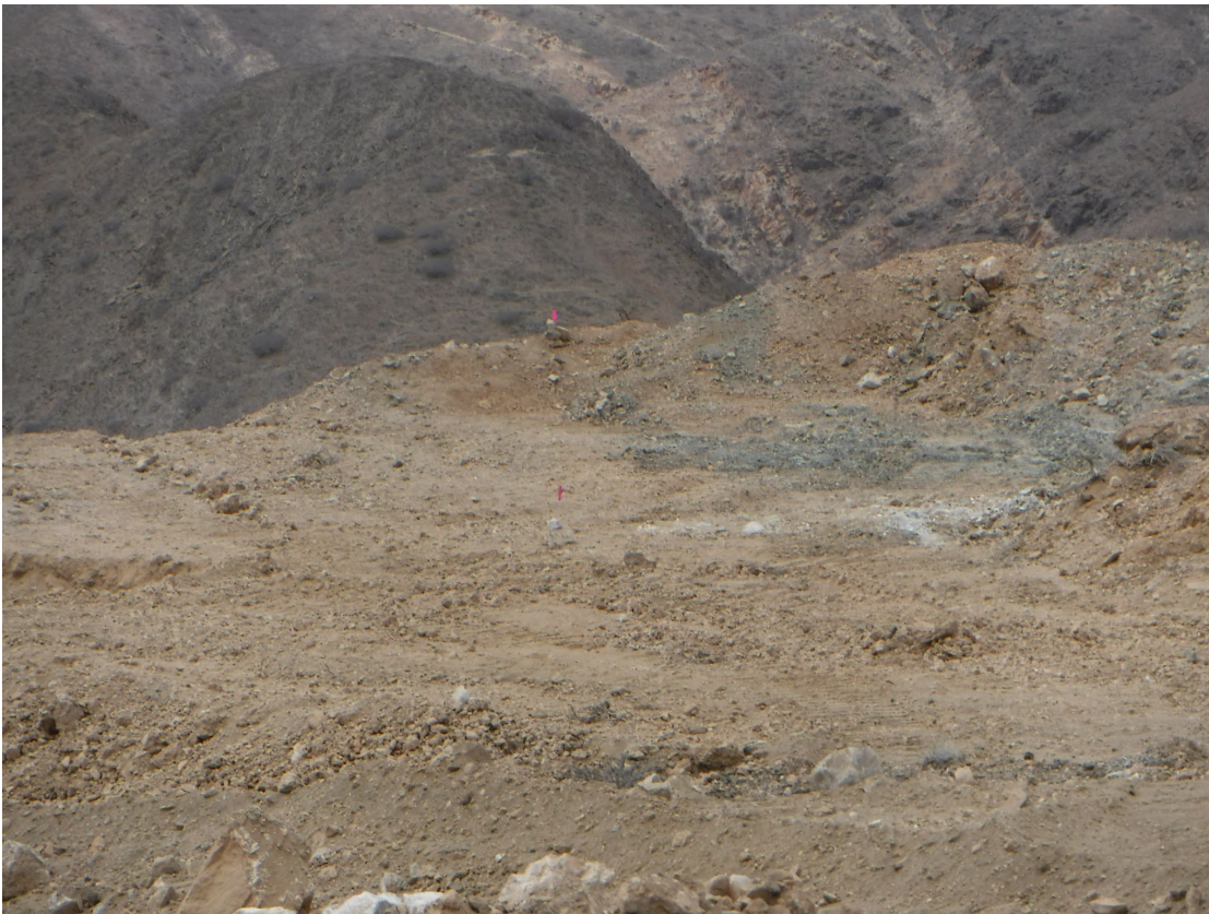
Figure 5: First drill-hole marked-up, with drill collar to be situated at pink pin-marker near the centre of the image, with hole to be drilled towards the distant pink pin-marker.
