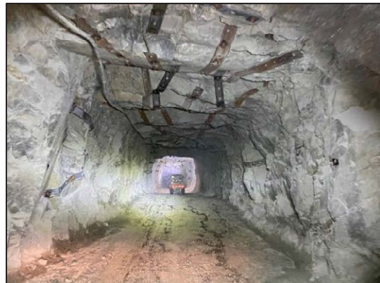
Underground intersection showing good ground conditions and existing services
