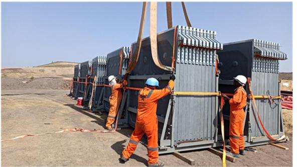
**Plates for pressure filter 2500 (Matec)**
