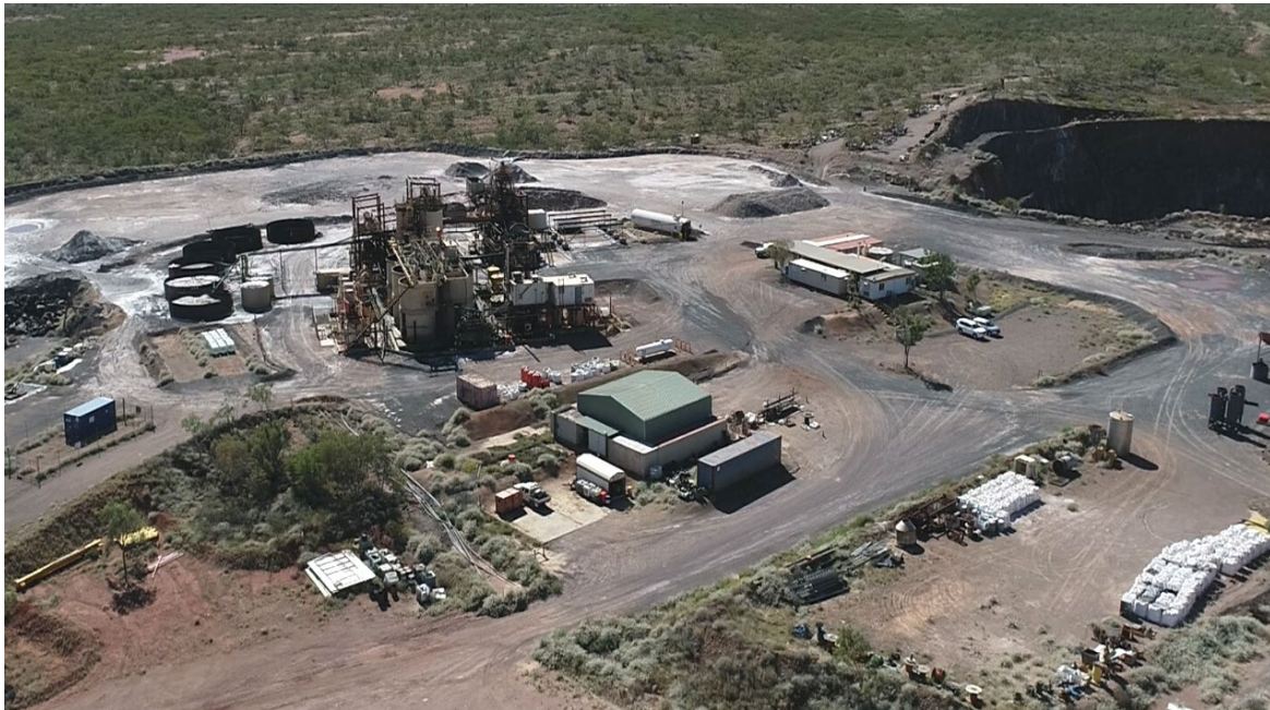
Image 5 - Lorena Processing Plant
