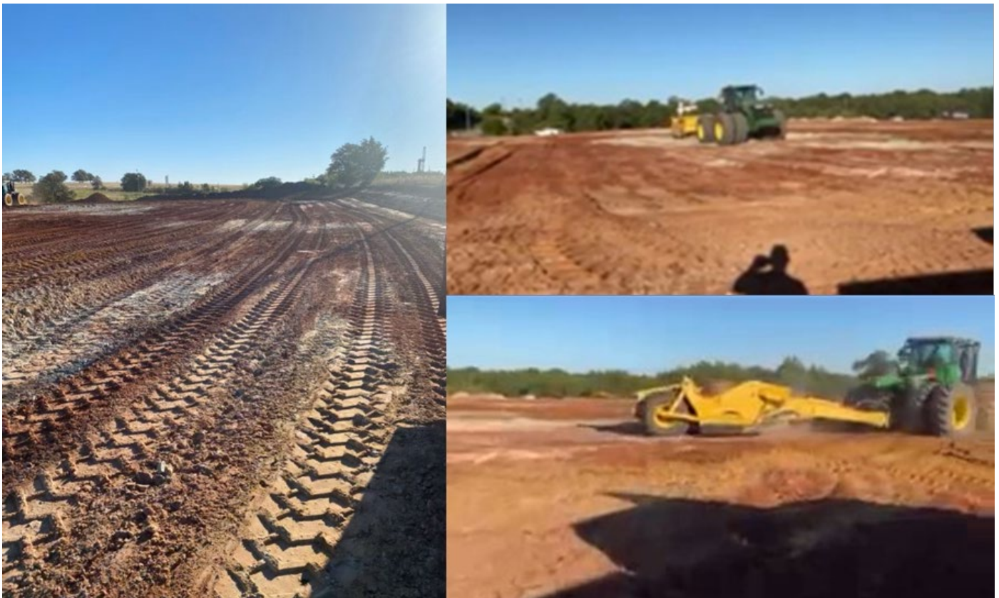
Figure 1. Construction of the all-weather pad for the Wolf Pack Well.
