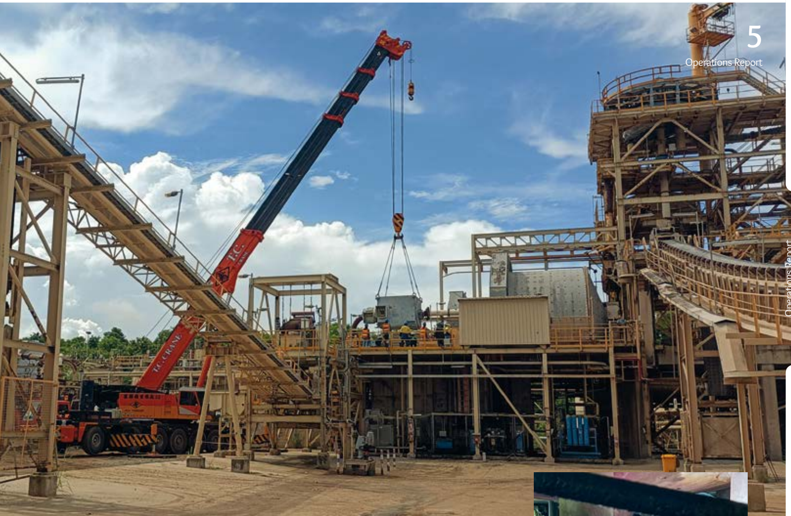
CR3 undertaking refurbishment works on Plant #2
