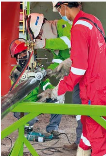
CR3 engineers machining replacement parts for Plant #2
