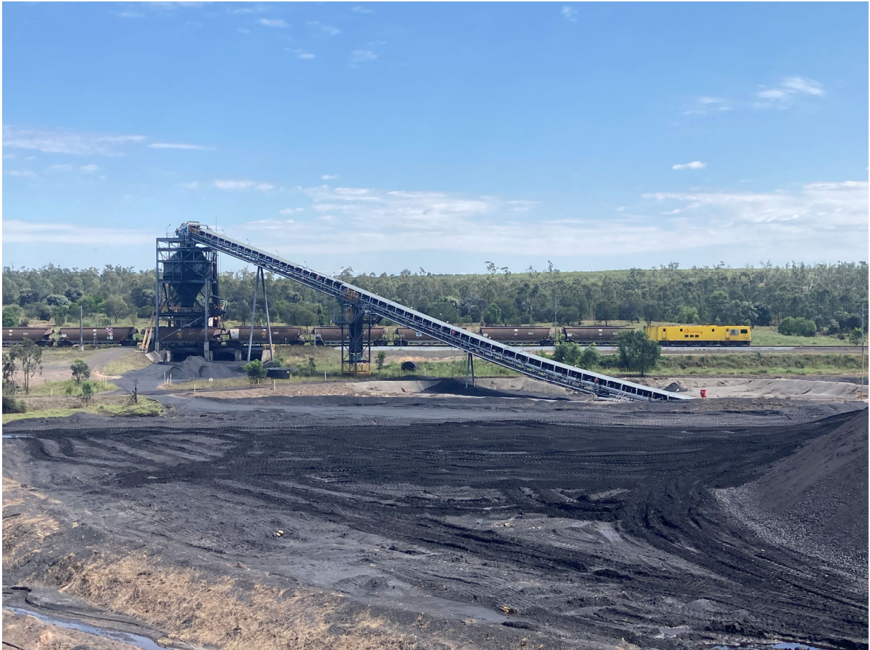
Figure 1: First coal being loaded from the Company's Broadmeadow East pit near Moranbah, Queensland.
