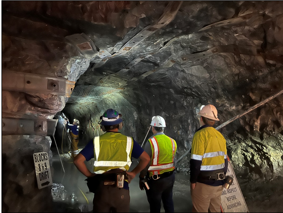
Photo 3 - Installation of ground support
