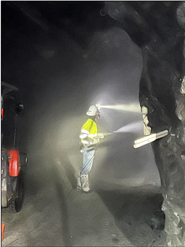
Photo 5 - Washing down underground walls in preparation for sampling and mapping
