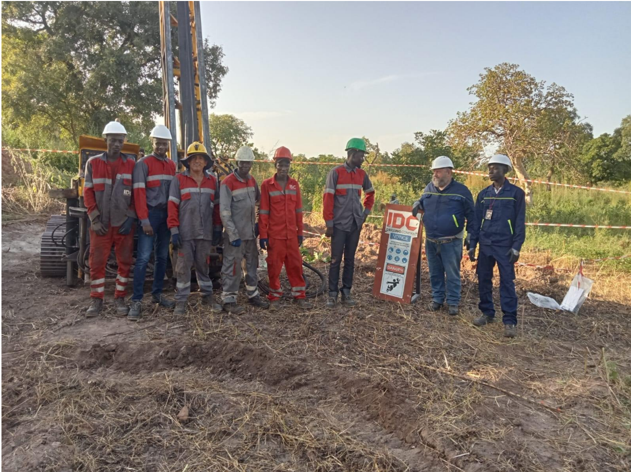
Figure 3: IDC drill rig and team, including members of Haranga's team onsite for commencement of drilling
