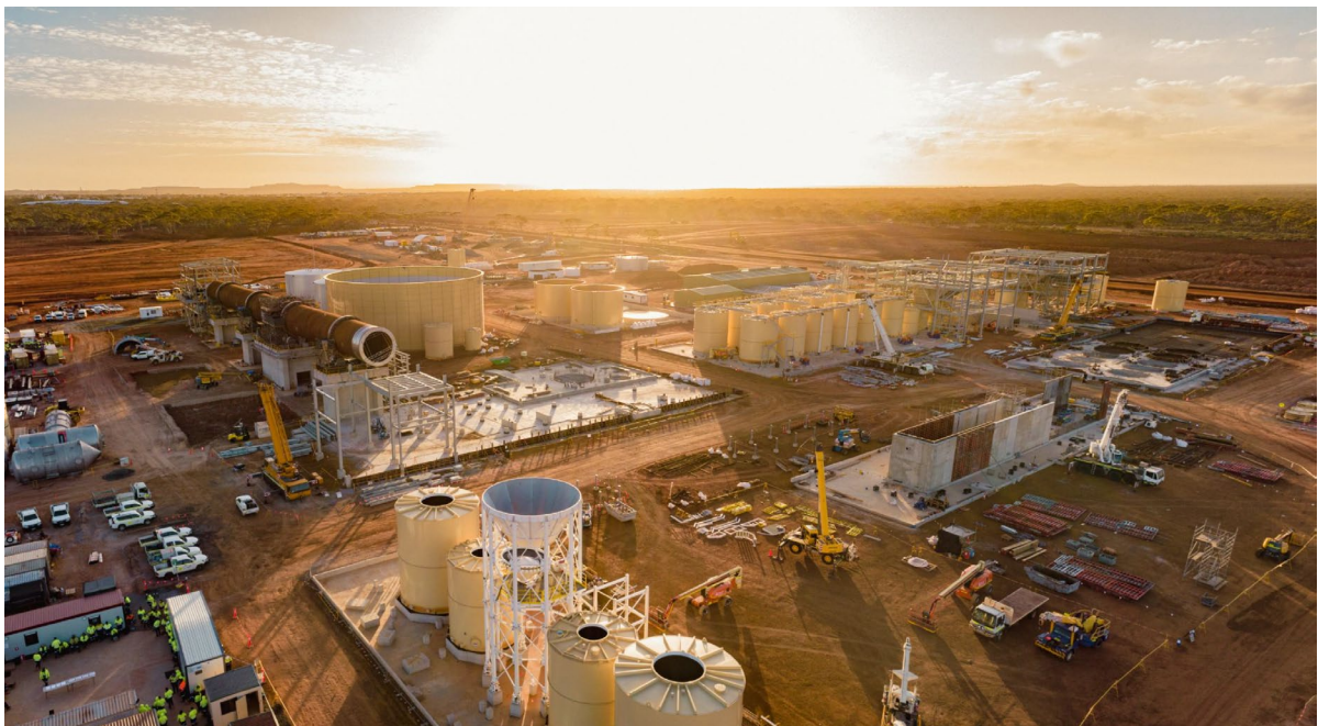
Aerial view of Kalgoorlie construction works looking south east, October 2022
