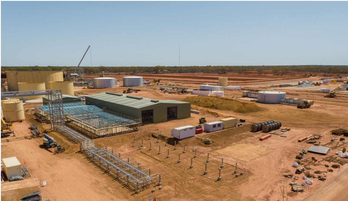
Workshop Warehouse complete and Control room and Maintenance Offices Progressing
