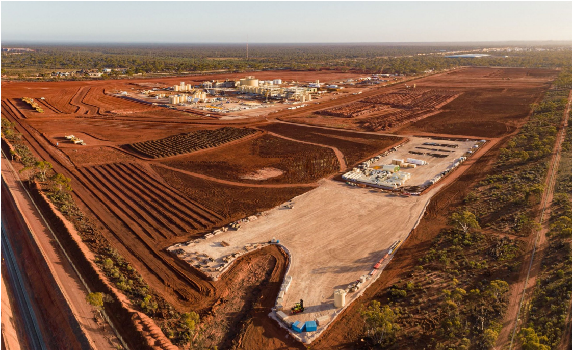
Byproduct Storage Facilities and Evaporation Ponds Construction Underway
