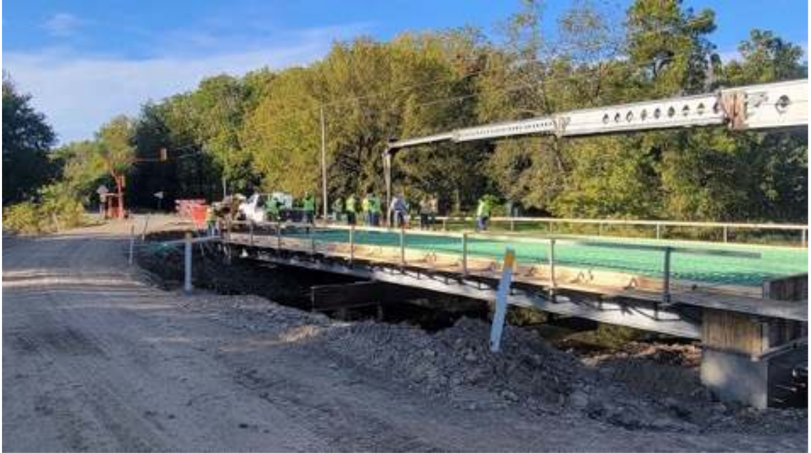
Figure 2. EdenCrete® bridge trial in Clinton County, Iowa
