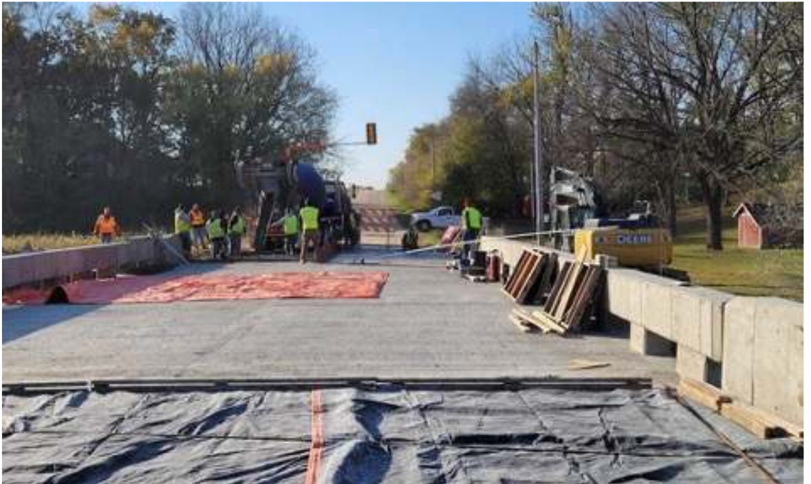
Figure 3. EdenCrete® bridge trial in Clinton County, Iowa
