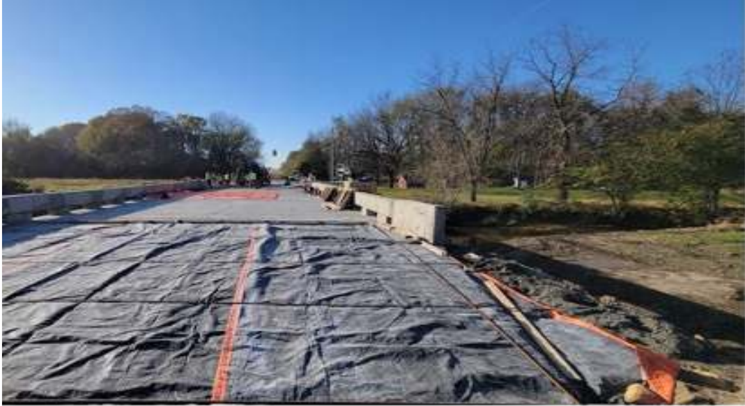
Figure 4. EdenCrete® bridge trial in Clinton County, Iowa
