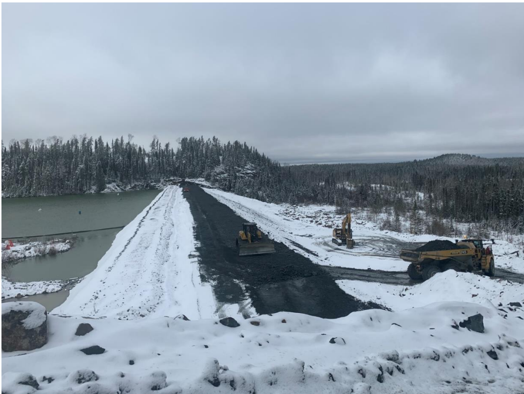
Figure 1: Sugar Zone tailings lift works
