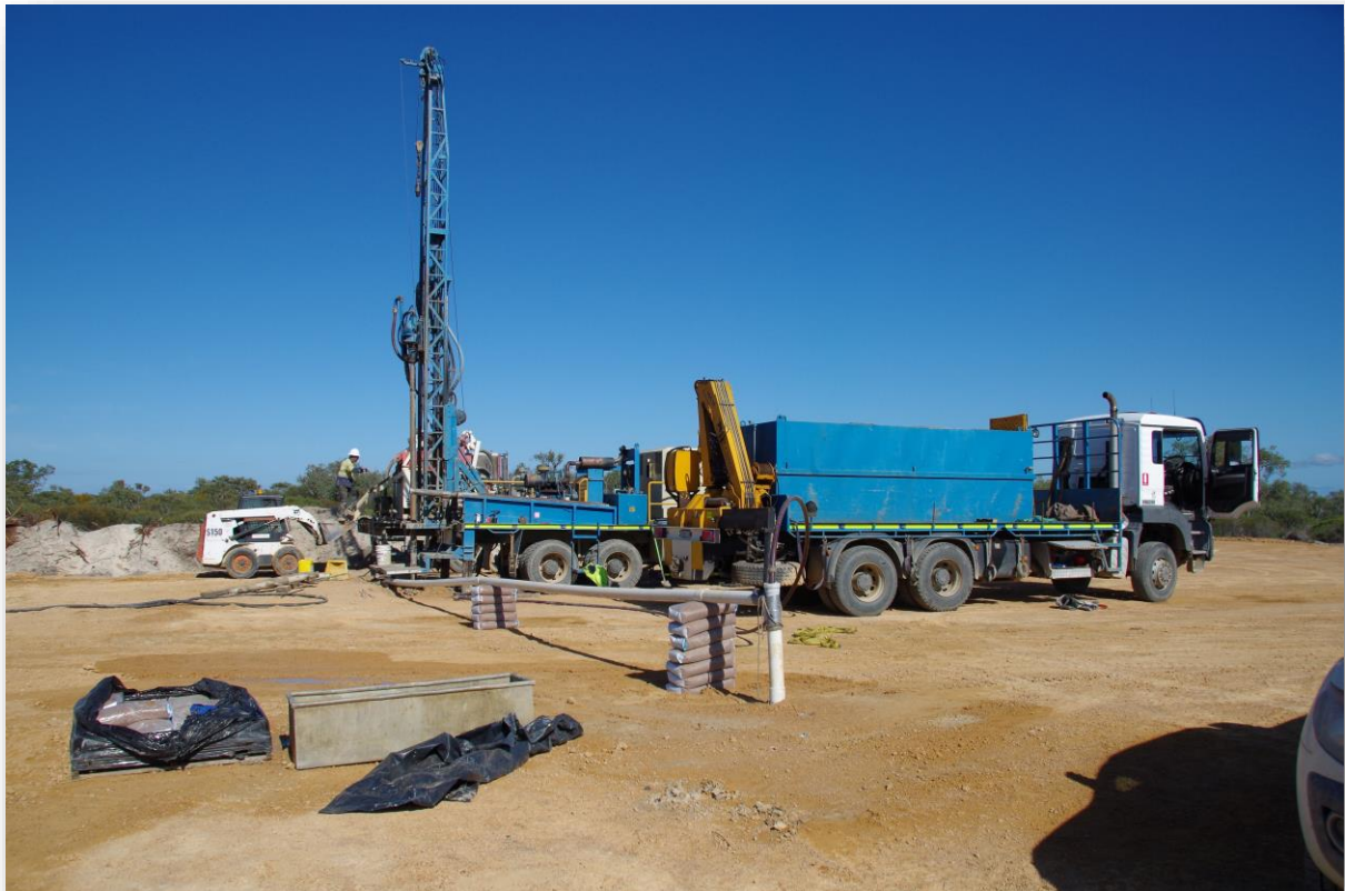
Figure 5: Water Bore Rig onsite
