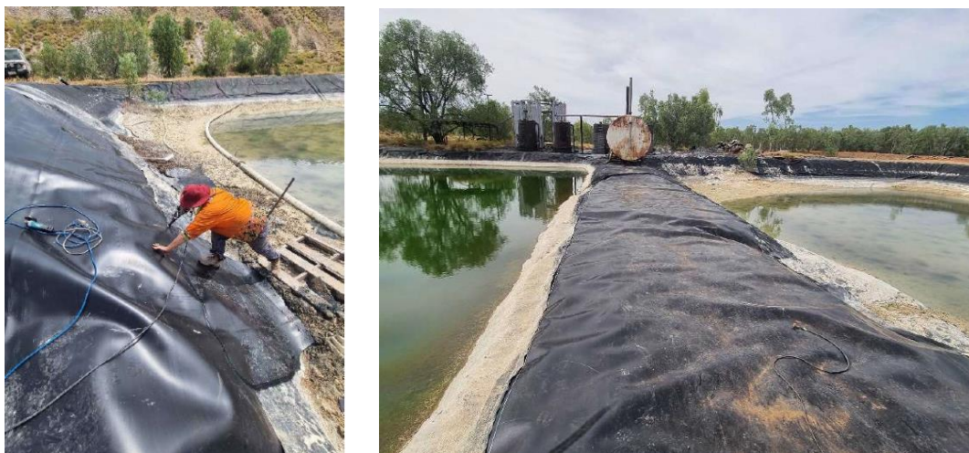
Figure 22: Repair works to HDPE liner at Yandan former process ponds
