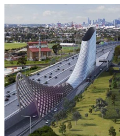
Westgate Tunnel Switchboards – Trivantage Manufacturing Over $10m
