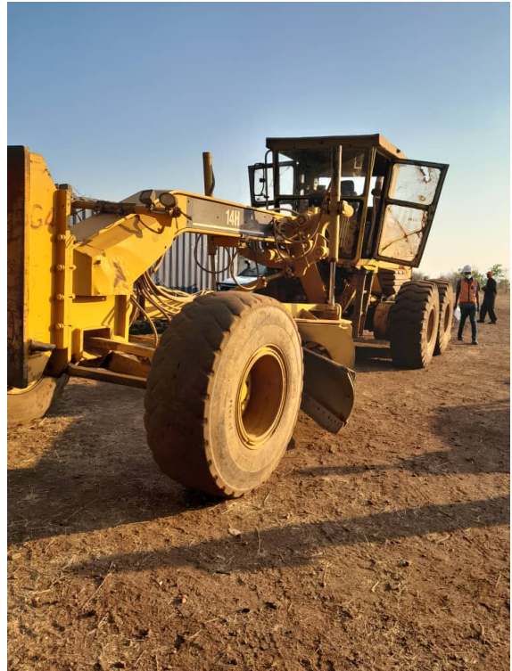
Grader on site maintaining access road
