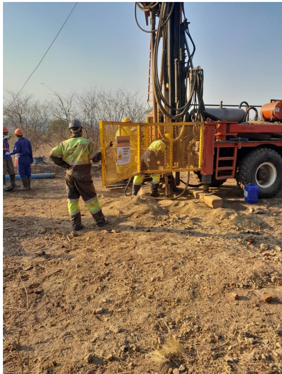
Drill hole preparation
