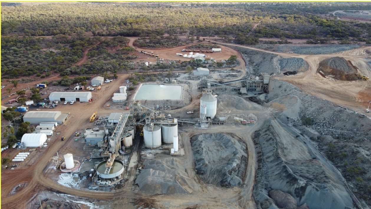
Figure 2 – 1.2Mtpa Processing Plant at Davyhurst
