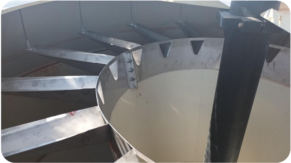
Trial radial froth launder installation in flotation cell 1
