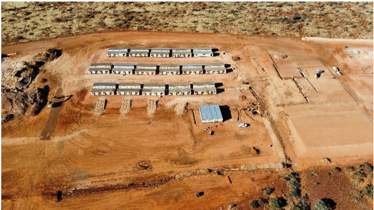
Figure. 1 Accommodation Village: Phase 1 with First 100 rooms installed in place.
