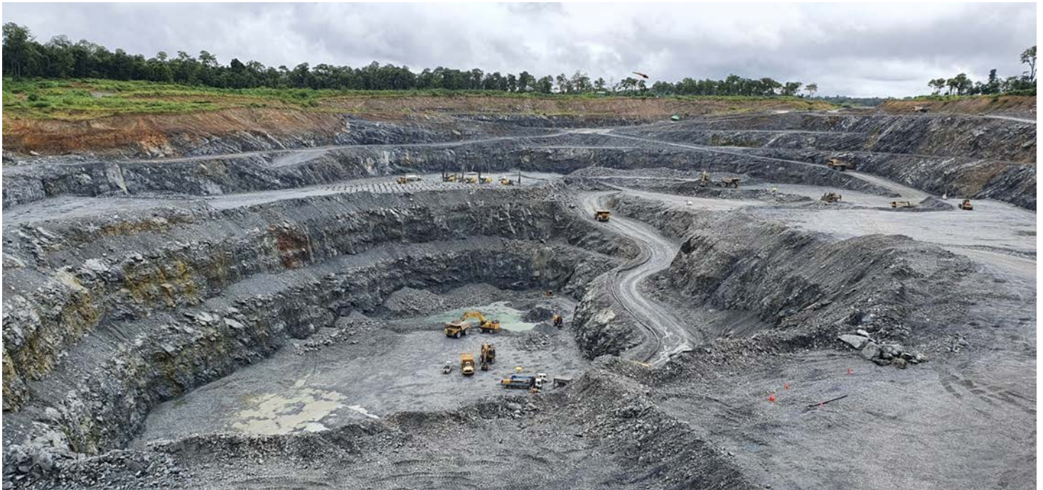
Figure 1 | Okvau Open Pit 20 September 2022 (nearing completion of wet season)
