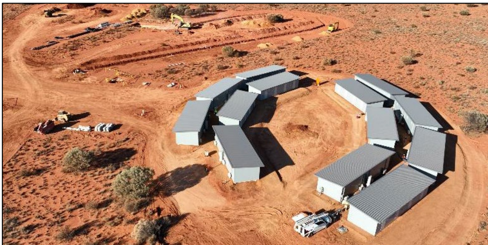
Figure 2: Accommodation Village building installation progress as at September quarter-end.
