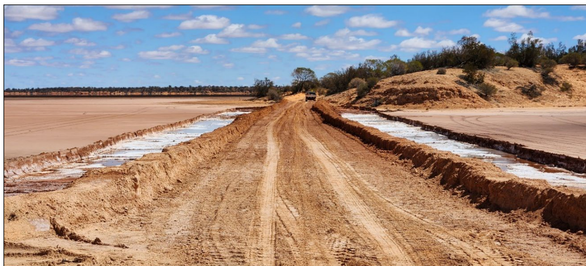
Figure 3: Causeway across lake surface to facilitate drilling campaign
