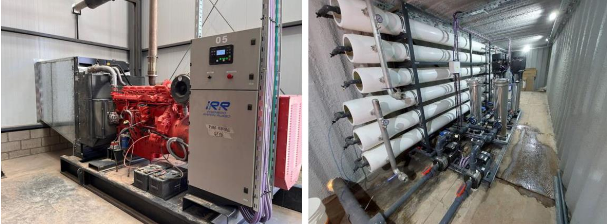
Figures 7-8. Rincon Lithium Project – 2,000tpa Operation Commissioning Works
