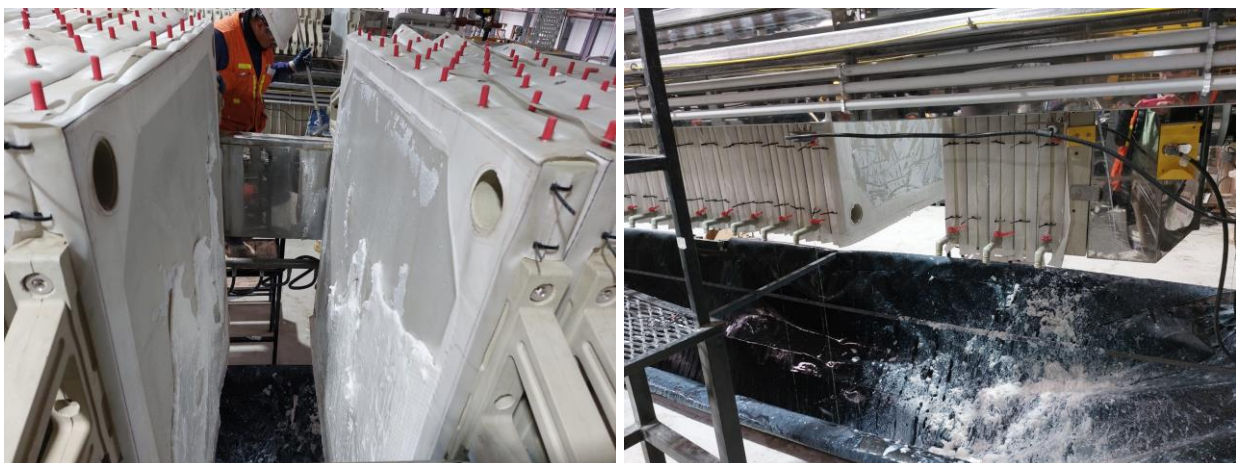
Figures 5-6. Rincon Lithium Project – 2,000tpa Operation Commissioning & Product Test-Works
