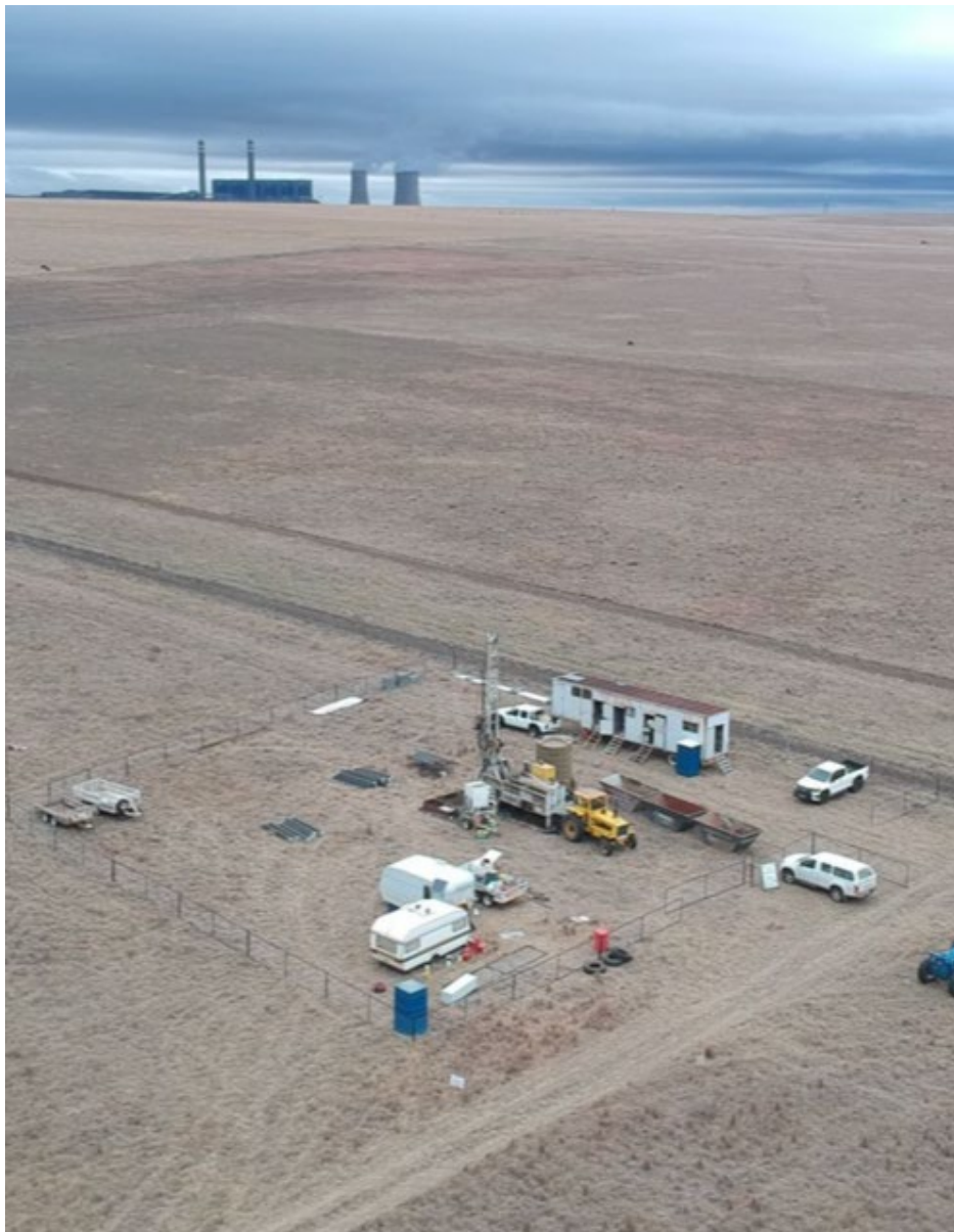
Figure 1: Core well 271-23C (previously KV-14C) being drilled with the Majuba Power station in the background
