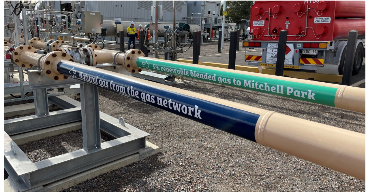
The HypSA Project in Tonsley, South Australia, is blending up to 5% Hydrogen into the local gas network
