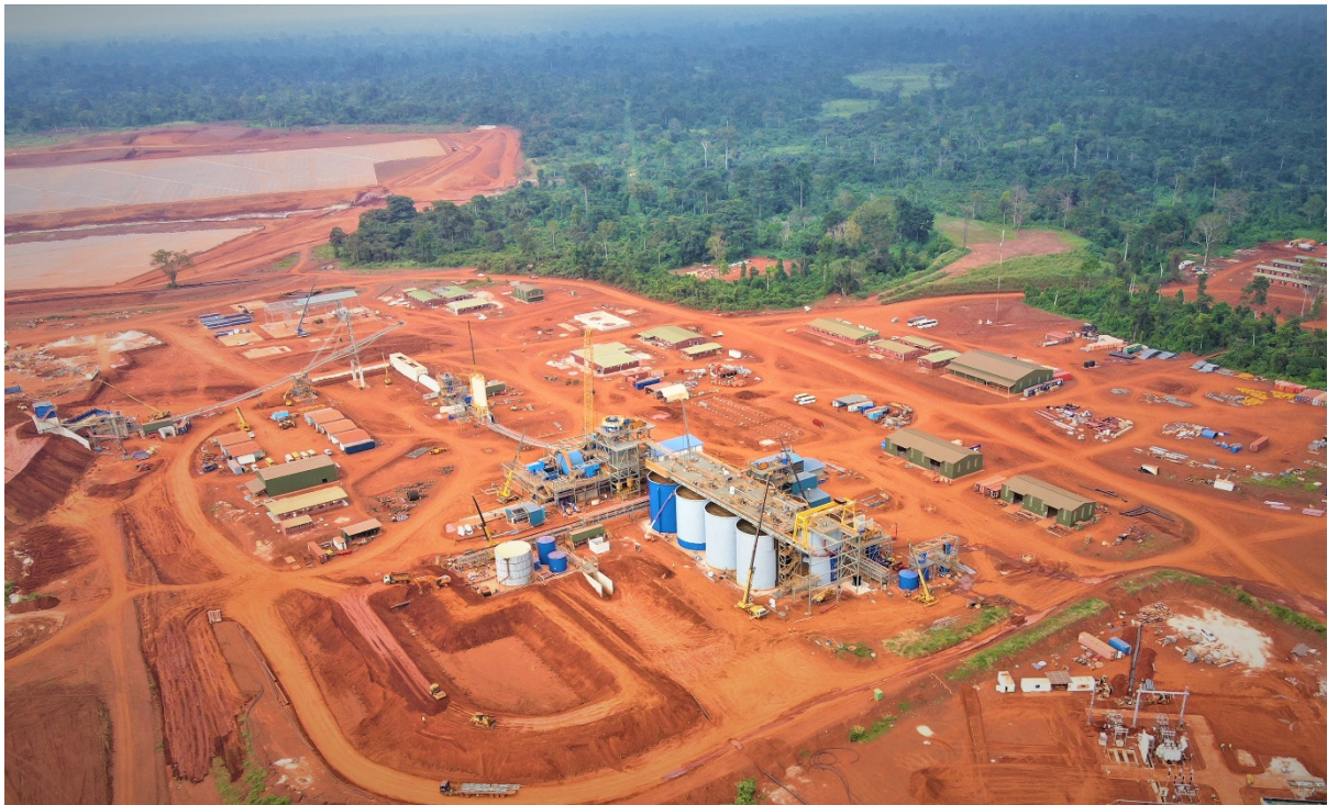
Figure 4: Abujar plant progress
