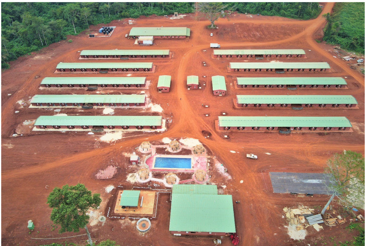
Figure 6: Accommodation camp and facilities
