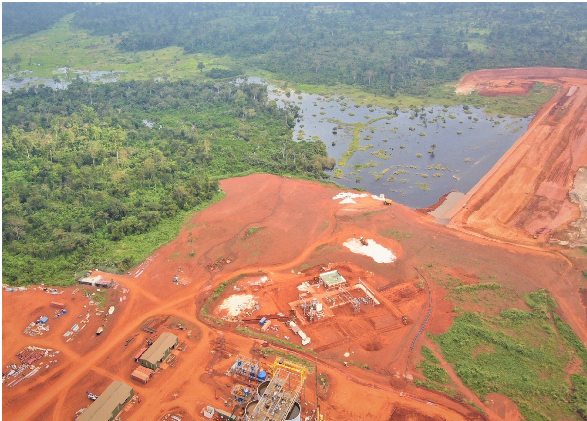
Figure 8: Water storage progress
