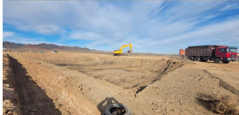
Pilot site construction
