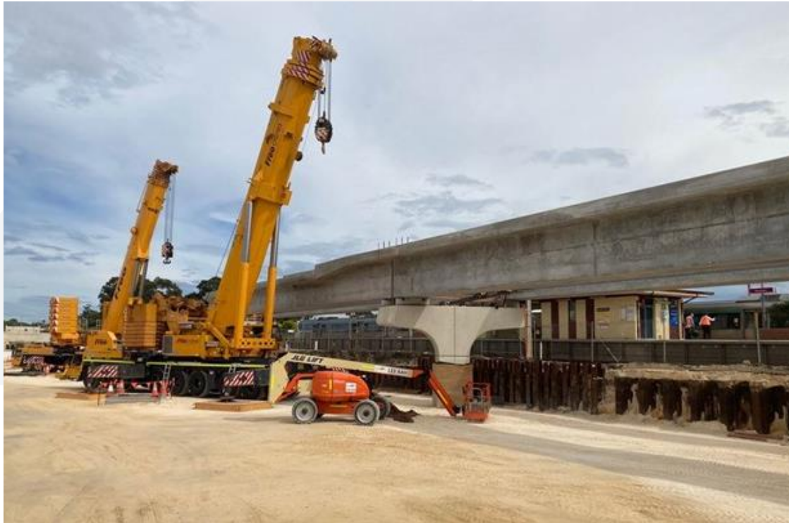
Beam Installations at Bayswater Train Station
