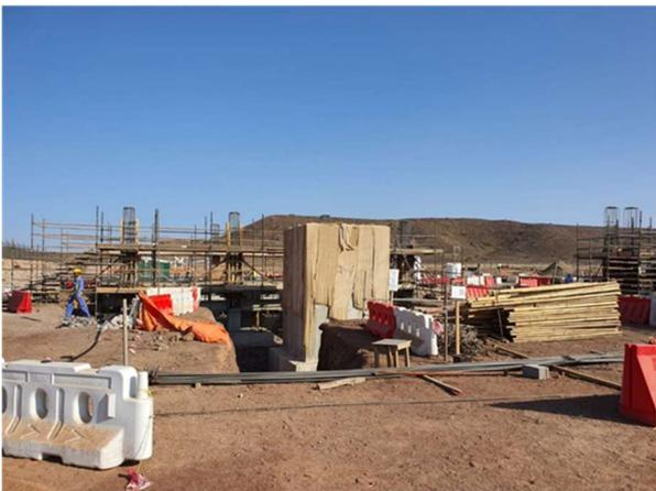
***Regrind mill foundation works***
