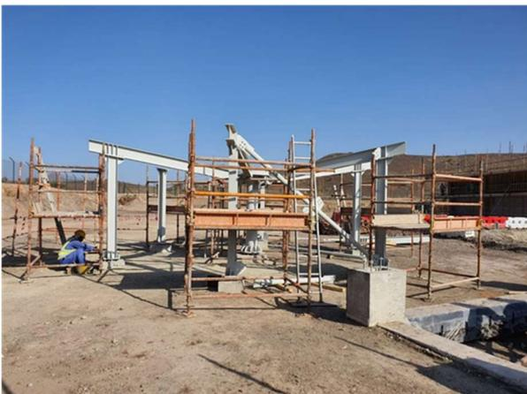
***Copper concentrate thickener erection in progress***
