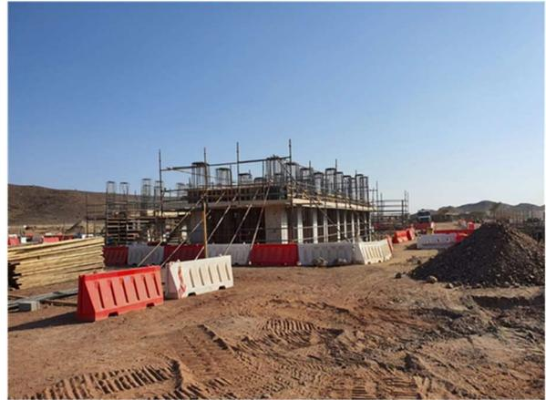
***Rougher flotation cell foundation works***
