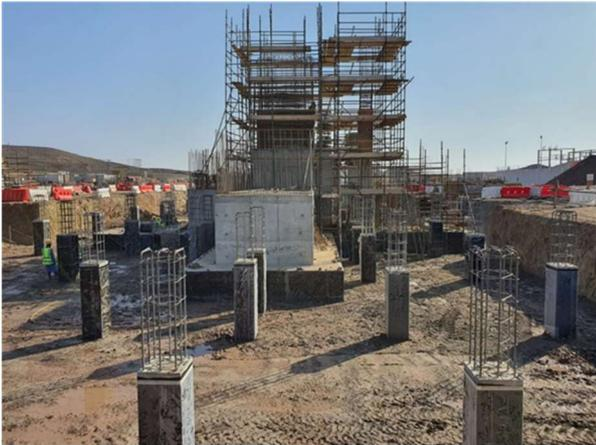
***Mill area platform column foundation works***
