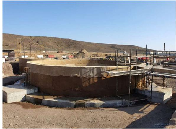
**Tailing filter tank foundation**
