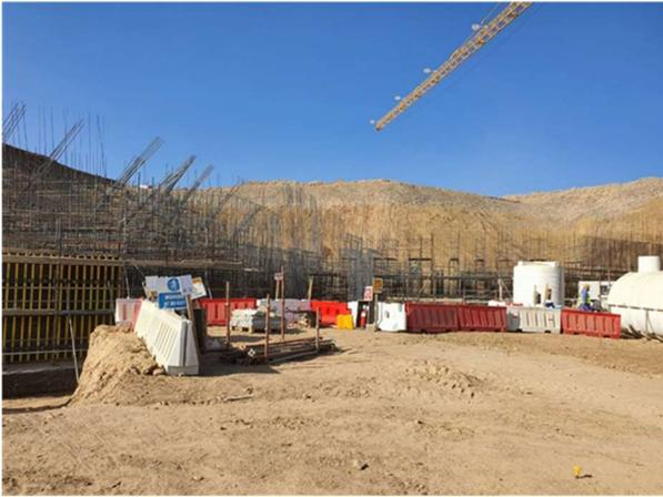
**Primary crusher retaining wall under construction**
