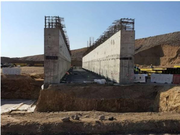
***Crushed ore stockpile side walls completed***
