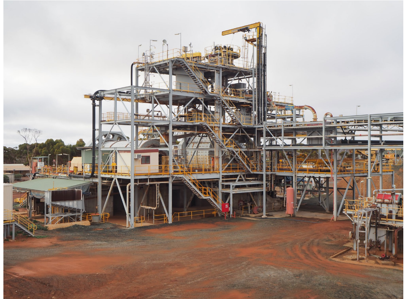
Black Swan Grinding Circuit and Flash Flotation
