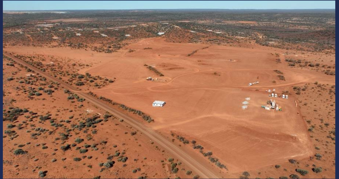
Plant Site cleared by a Tjiwarl contracting business
