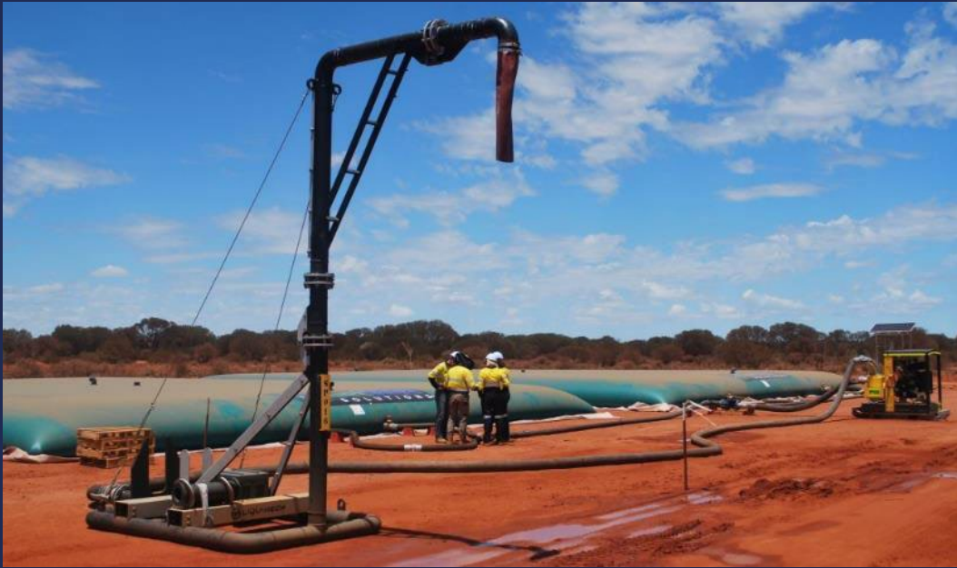
Construction water bladders and standpipe
