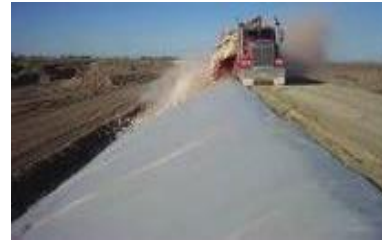
POND 5 EMBANKMENT TRIAL
