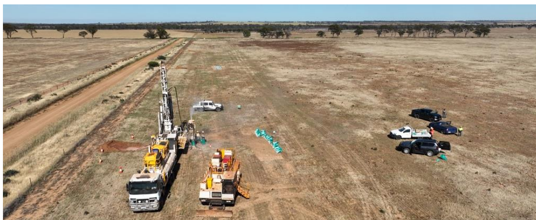
Figure 1: Strike Drilling Morooka based Aircore rig on site at Hines Hill REE Project
