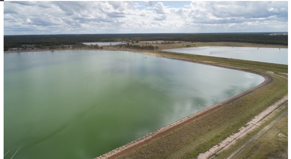
Waste brine ponds from coal seam gas production in Queensland, Australia.
