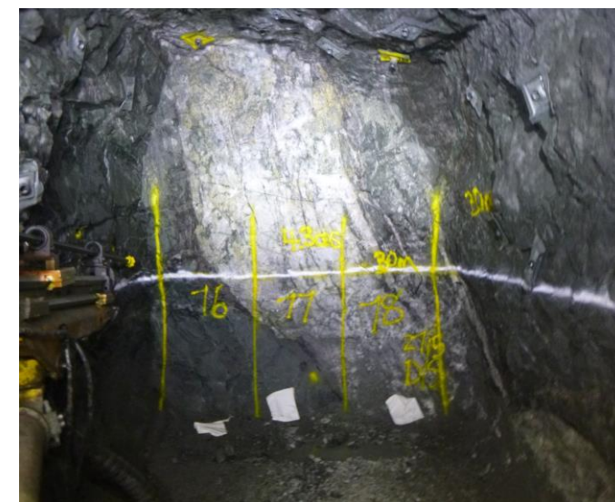
4.3 Level ore drive face 1
