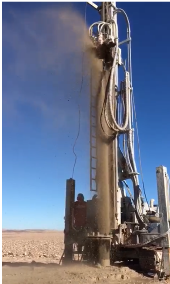
Figure 3: High pressure brine encountered in drilling
