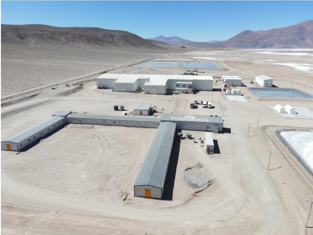
Figure 10. Rincon Lithium Project – 2,000tpa Operations Site
