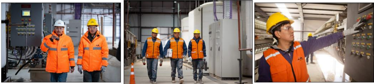
Figures 1-3. Rincon Lithium Project – 2,000tpa Operation Commissioning Works
