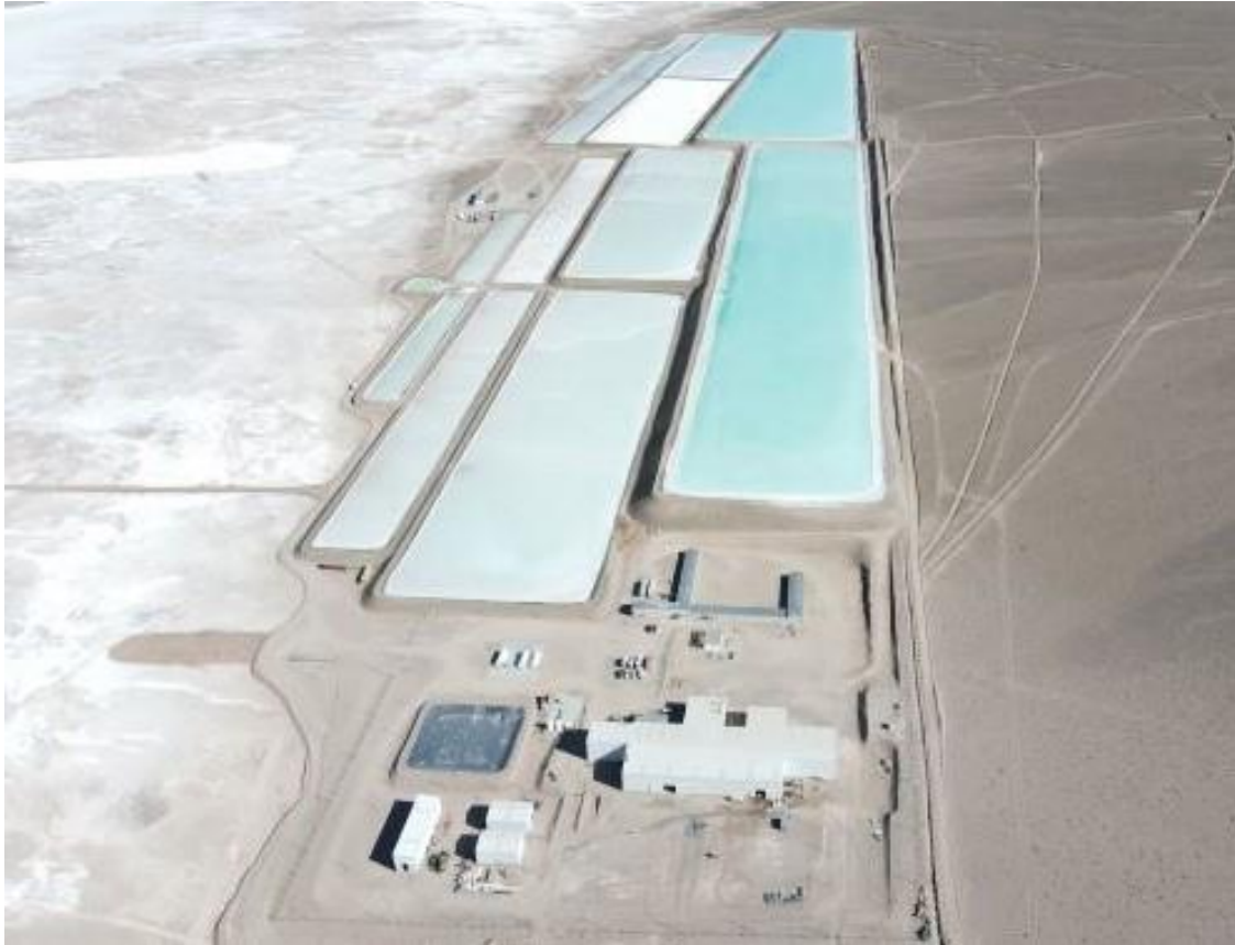
Figure 4. Rincon Lithium Project – 2,000tpa Operations Site
