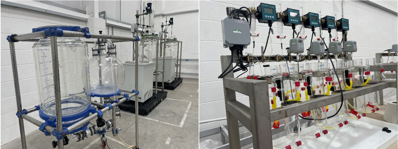
Figure 8: Process reactors and additional mixer-settlers delivered for the magnet recycling demonstration plant.
