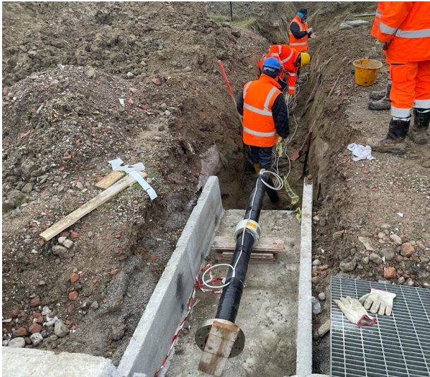
Anode installation
