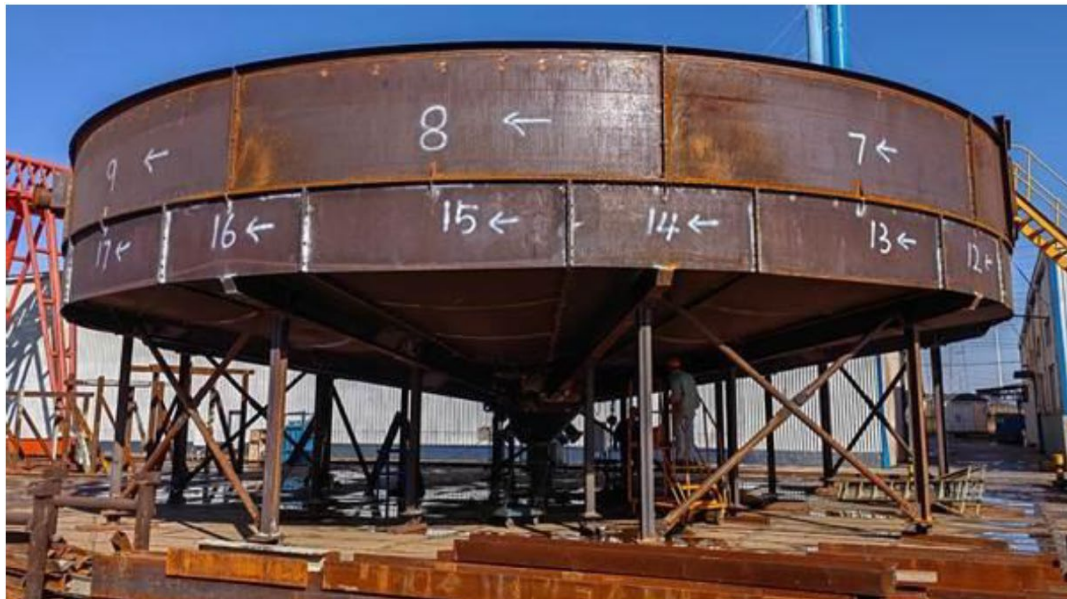
Figure 11: Thickener trial construction at factory
