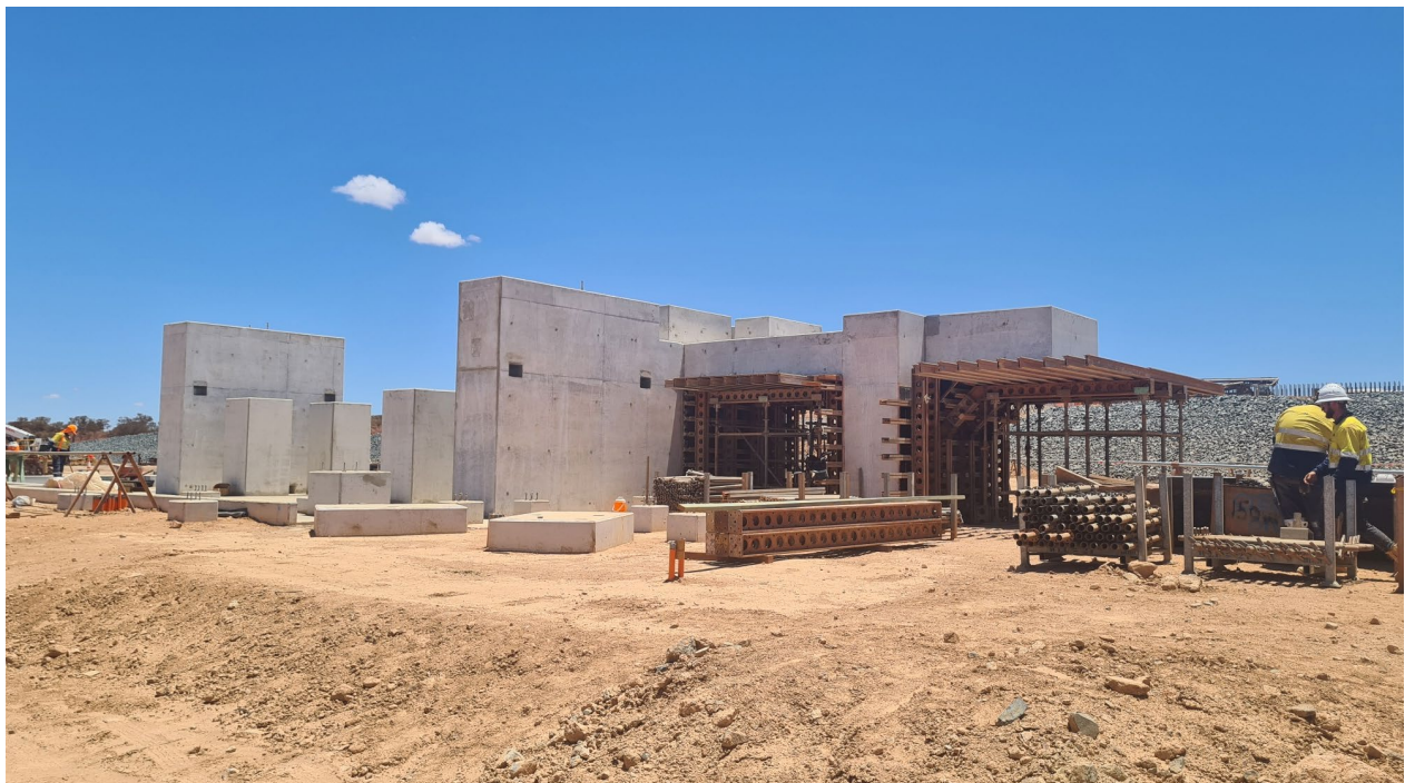
Figure 9: Close up of ball mill foundations
