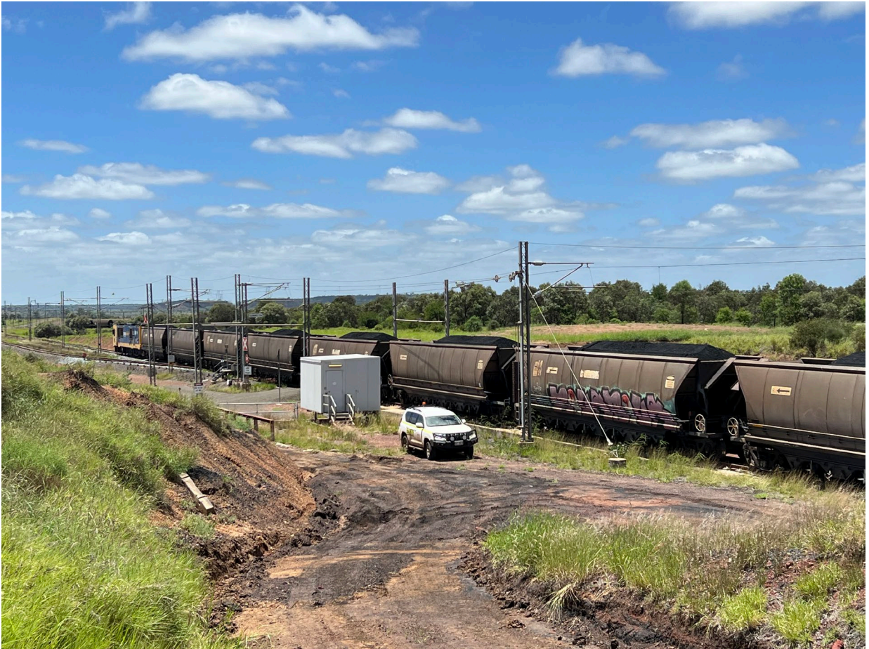
Figure 1: Bowen's first train loaded through its refurbished Mallowa TLO.
