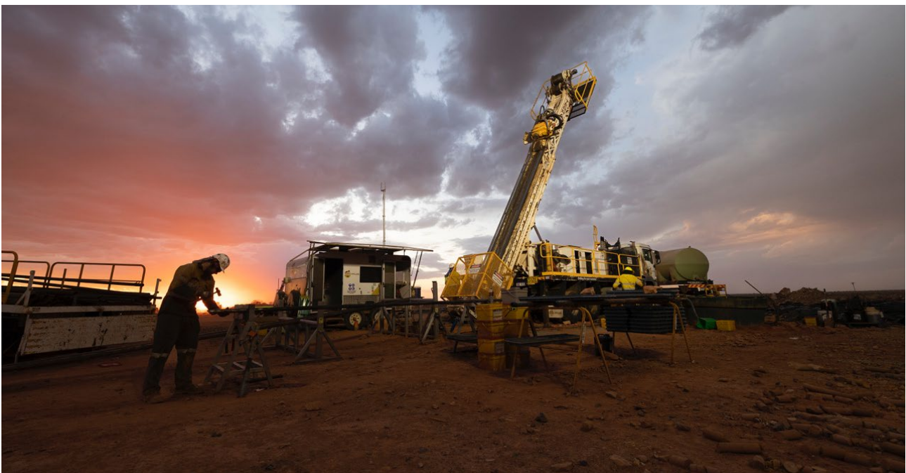
Figure 1: Drilling at Coyote Gold Operation in November 2022
