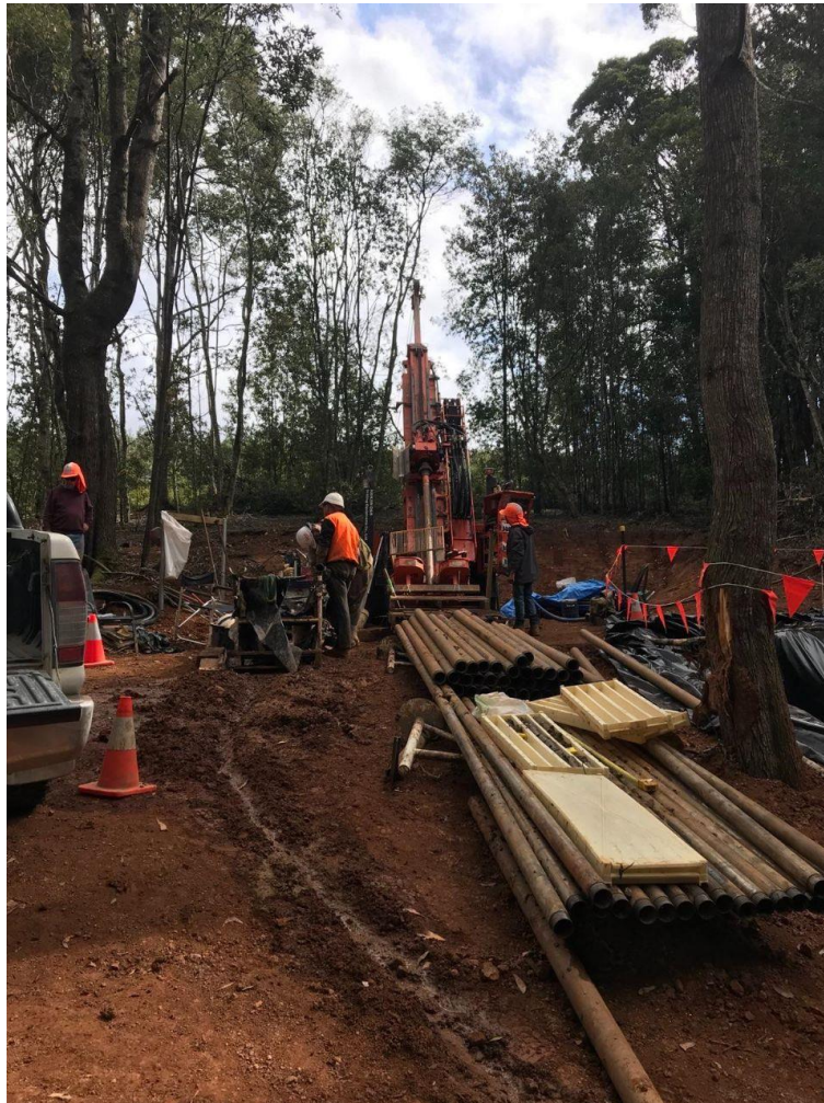
Figure 1: Drill on location at 22RRD-003
