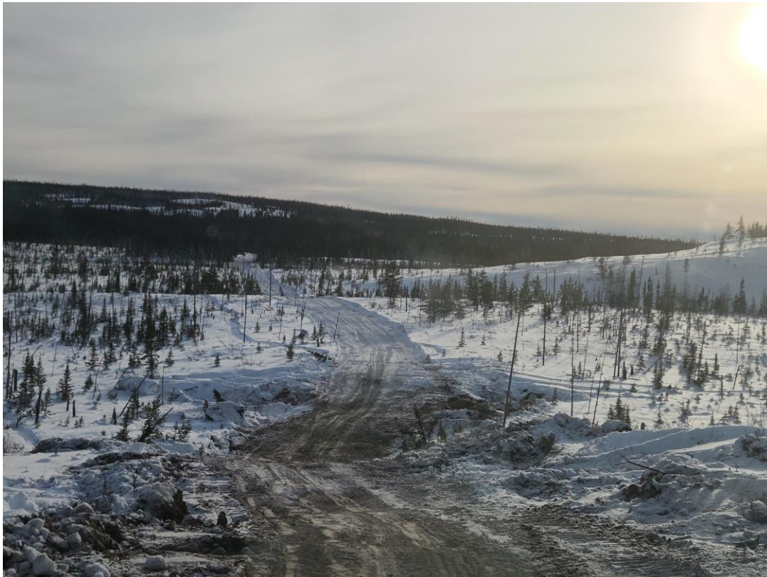
Figure 1: Segment of winter road extending from the Trans-Taiga Road to the drill area at CV5
