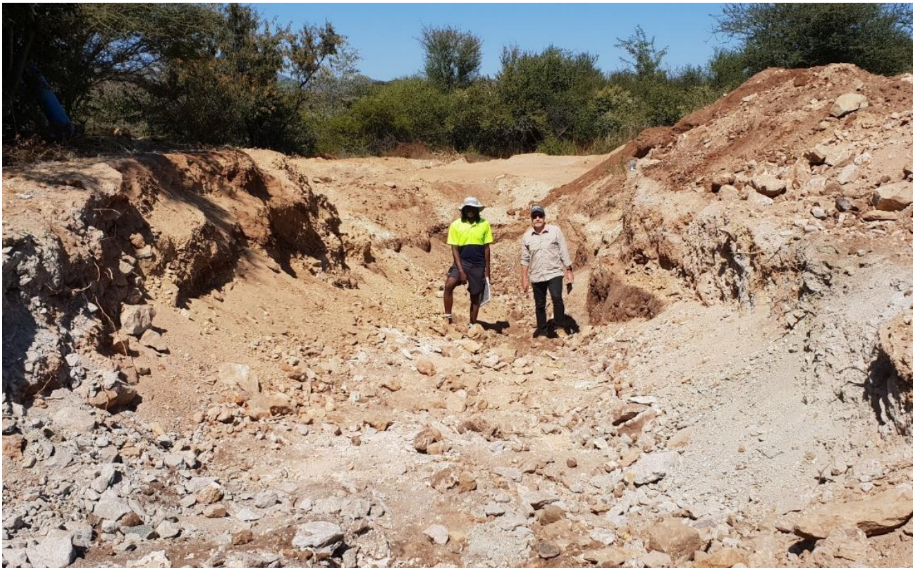
Image 3: Nosib Project bulk sample excavation for metallurgical testwork (geologist and CEO for scale).
