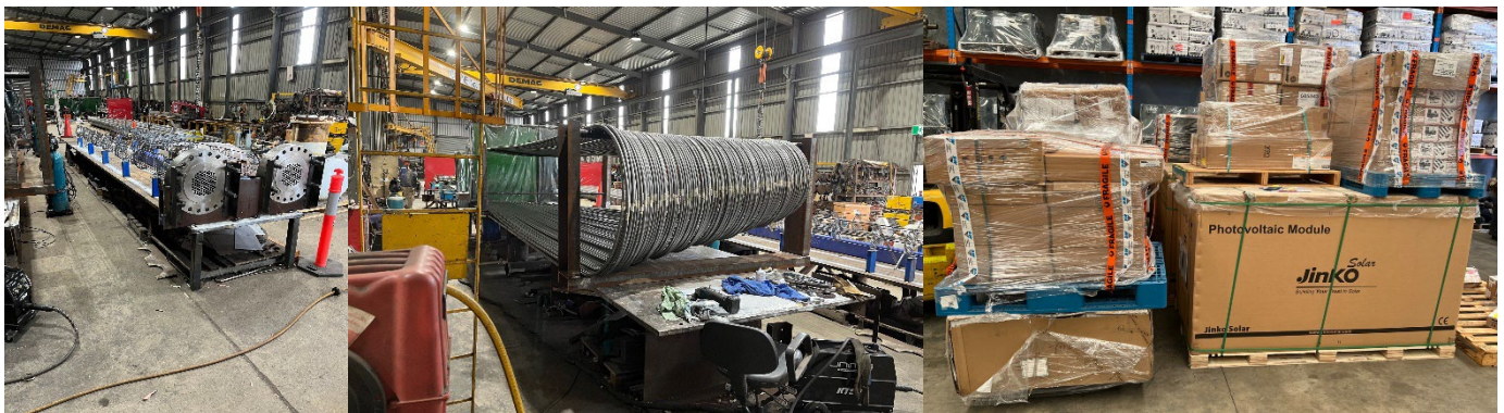
Above: Fabrication of Heat Exchanger for Walyering upstream facility and arrival of solar package to power the facility
