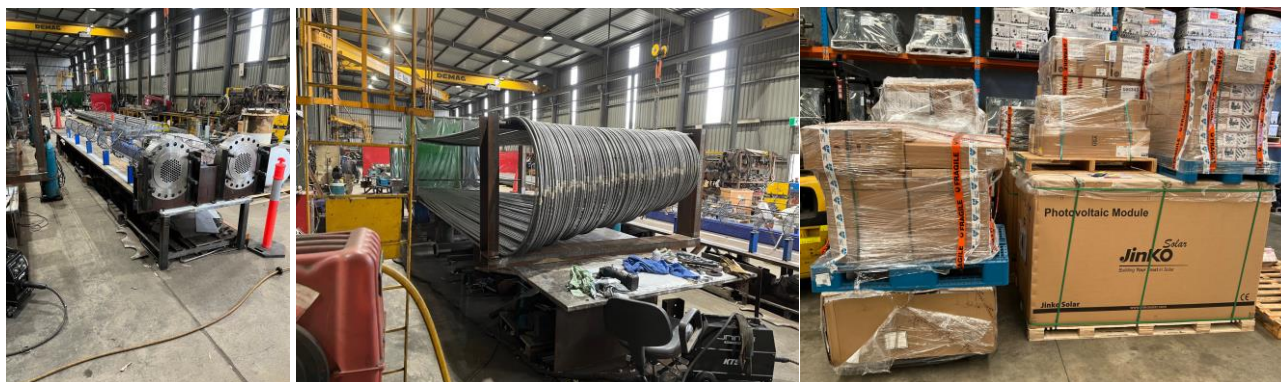
Above: Fabrication of Heat Exchanger for Walyering upstream facility and arrival of solar package to power the facility
