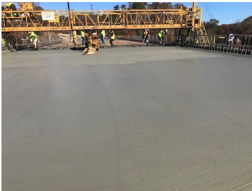
Figure 1. Little River bridge trial- showing freshly installed concrete
