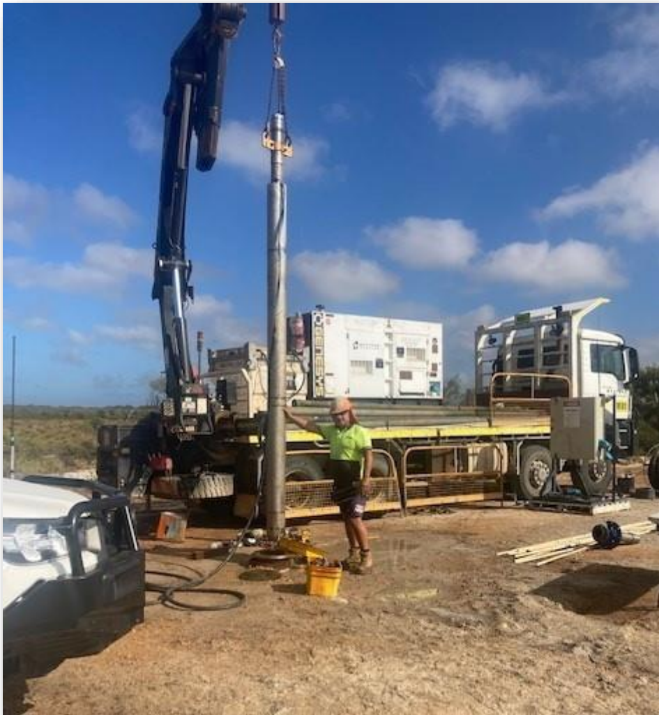
Figure 2: Bore testing equipment
