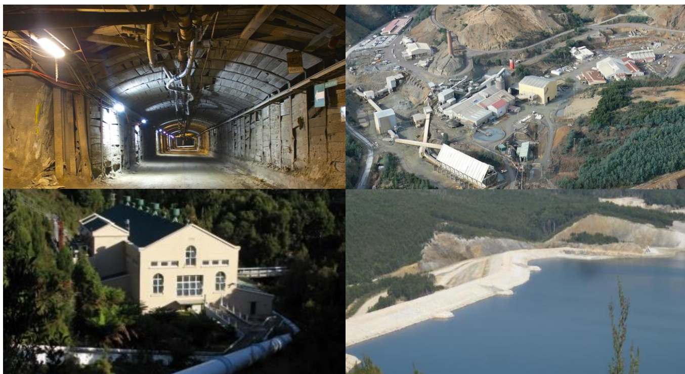
Figure 6 – Existing site infrastructure, clockwise from top left: underground workings, surface infrastructure, 100Mt capacity tailings dam, hydroelectric power station
